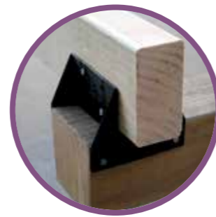
The positive connection between joist and bearer
